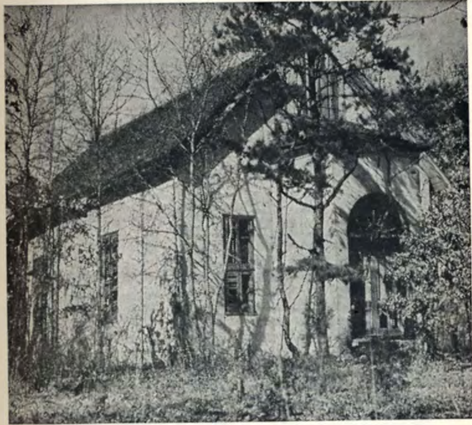
SCHOOL CHAPEL, LATER PRESBYTERIAN CHURCH —This structure, built in 1854 from some of the materials in the original Cokesbury Conference School, was used as the school chapel for a number of years. About 1876 it was acquired by a group of Presbyterians in Cokesbury and the building served as a Presbyterian church until the congregation in that community became too small to support a church.
