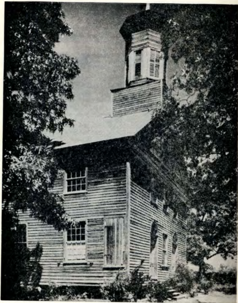
COKESBURY METHODIST CHURCH , built in 1837, was the central institution of the village, for the community has been described as "Methodist from center to circumference". This historic old structure was torn down in 1952 because it was badly in need of repair, and a new church building was erected on the same site. (Photo by Carl Julien).
