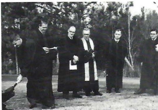
Ground Breaking for the New Educational building.
